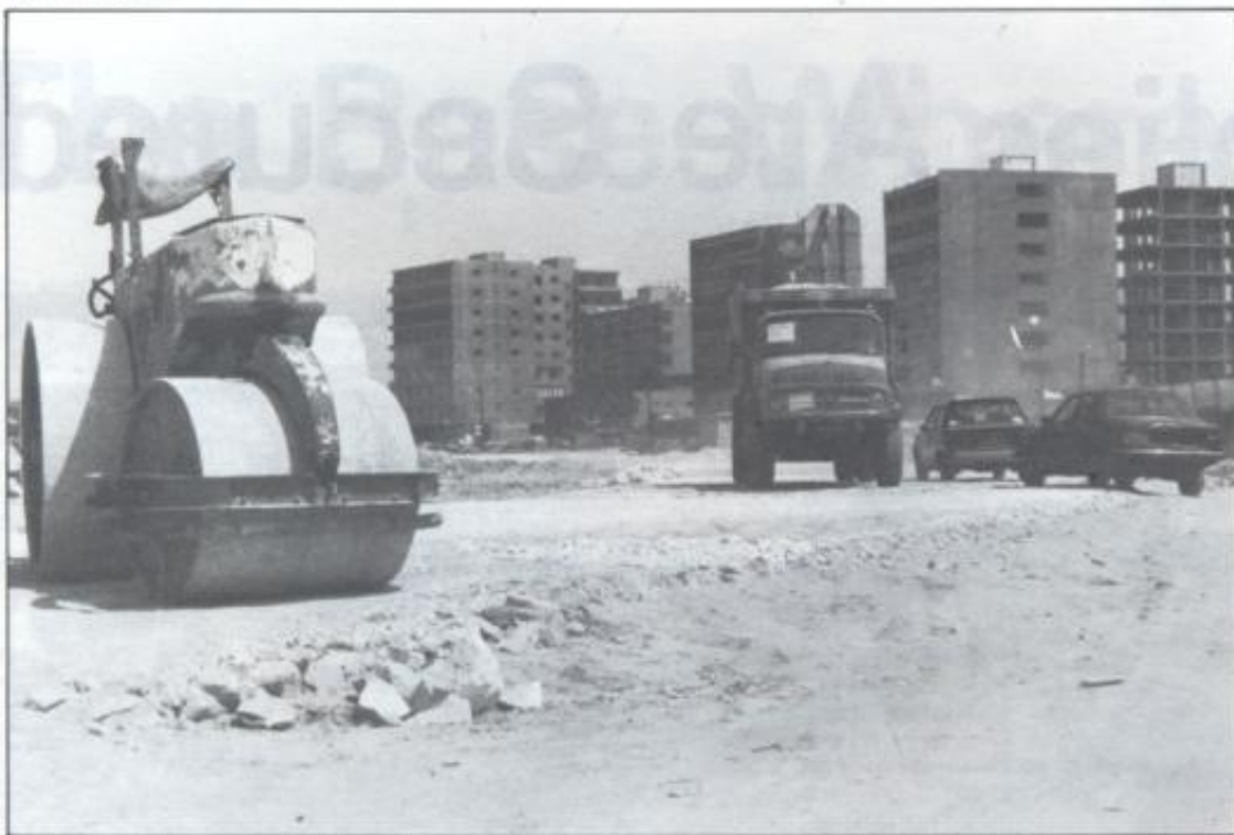
The road passing Tyre Log Base and leading to the harbour is now being reconstructed. This will provide better access route to the harbour than before.
