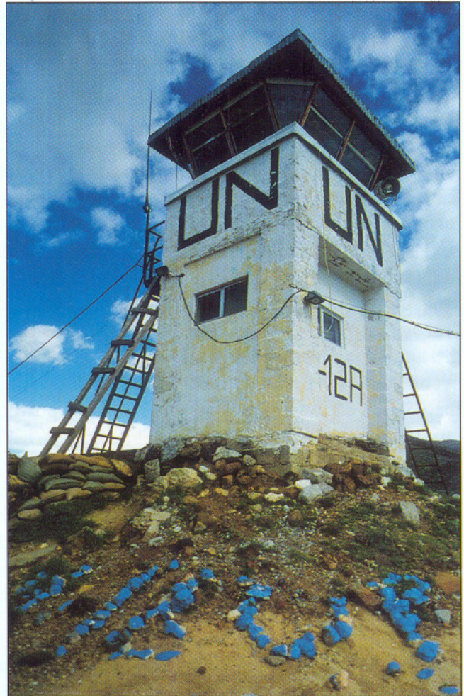
Constructed in XXVIII and still standing!
