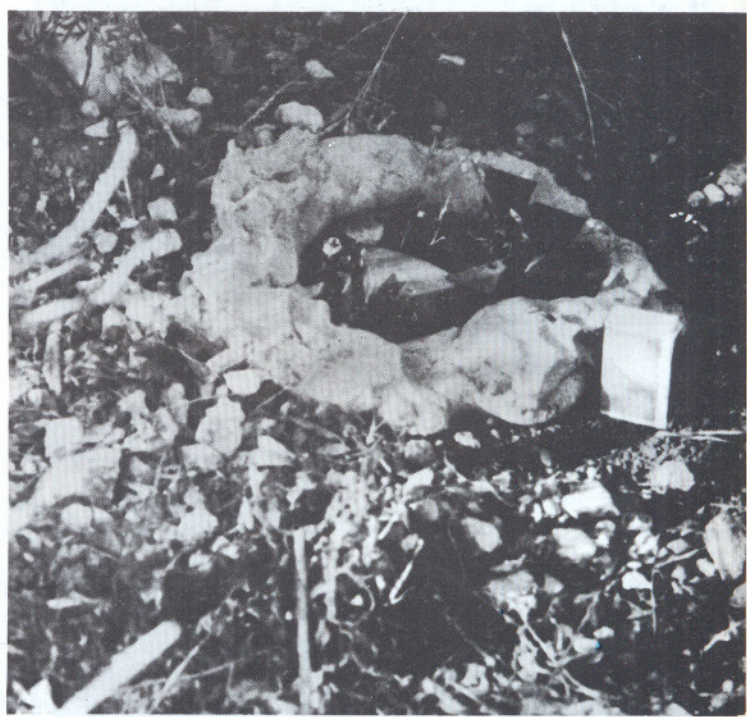
To livsfarlige clusters klargjort for sprengning.
